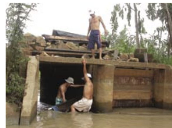
Managing sluice gates in TCNP. Photo: Tram Chim National Park
