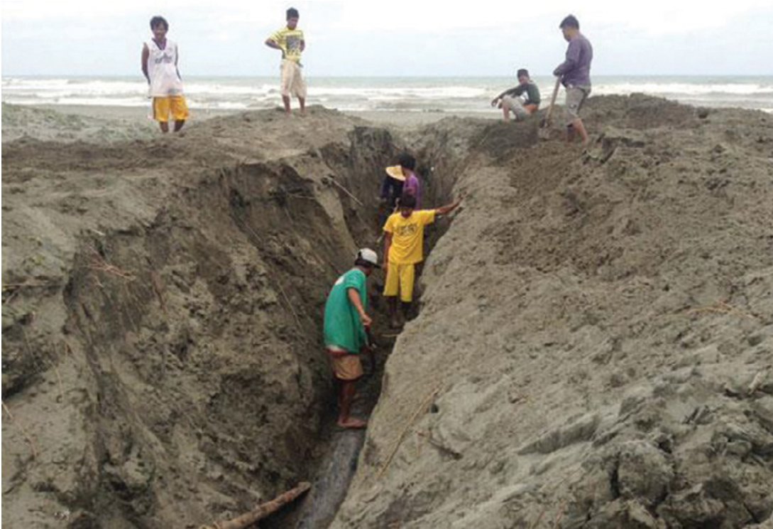
Residents of Punta village in Aparri, Cagayan try to remove a pipe abandoned by a black sand mining firm. Image from: Charlie Lagasca
