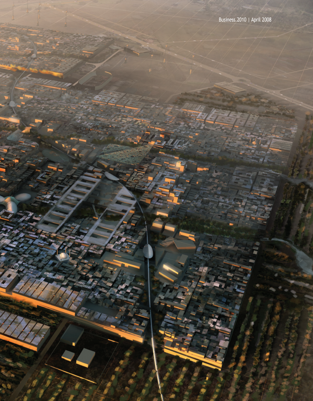
The Masdar City Master Plan in Abu Dhabi: The six square kilometre city, designed by Foster and Partner for the Abu Dhabi Future Energy Company, is to house an eventual 50,000 people. © Copyright Foster and Partners
