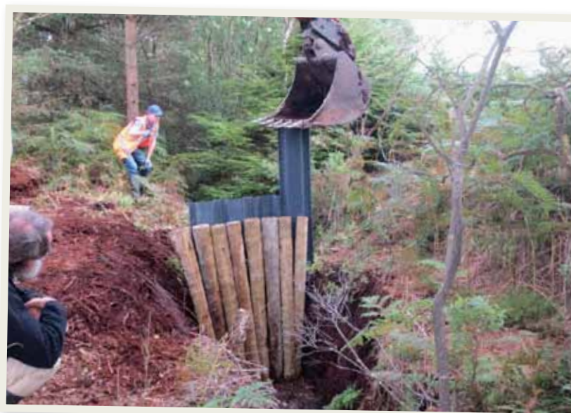
⬆ Drain blocking on Raised bog (Maurice Eakin)
