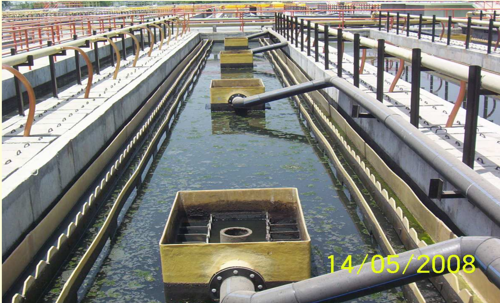
UASB Reactors
