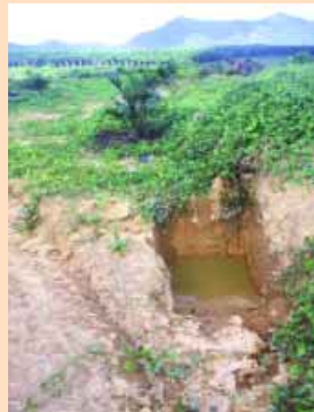
> During periods of heavy rainfall silt pits and roadside soakaways retain water and soil run-off
