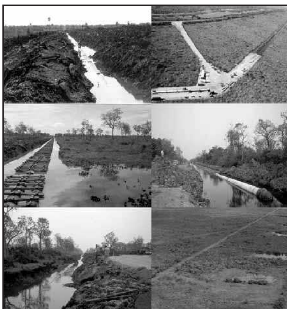
Shown in sequence, from left to right, top to bottom: the excavated trenches, platforms, pipe sections with floaters, pipes placed in trench, flooded trench, and current view of the ROW in the Pantanal.
