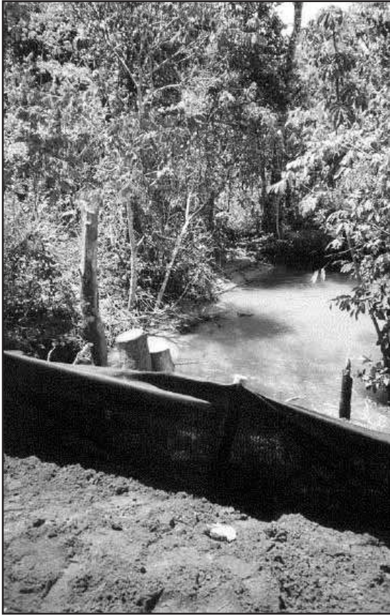
Sheet piling in conventional river crossings
