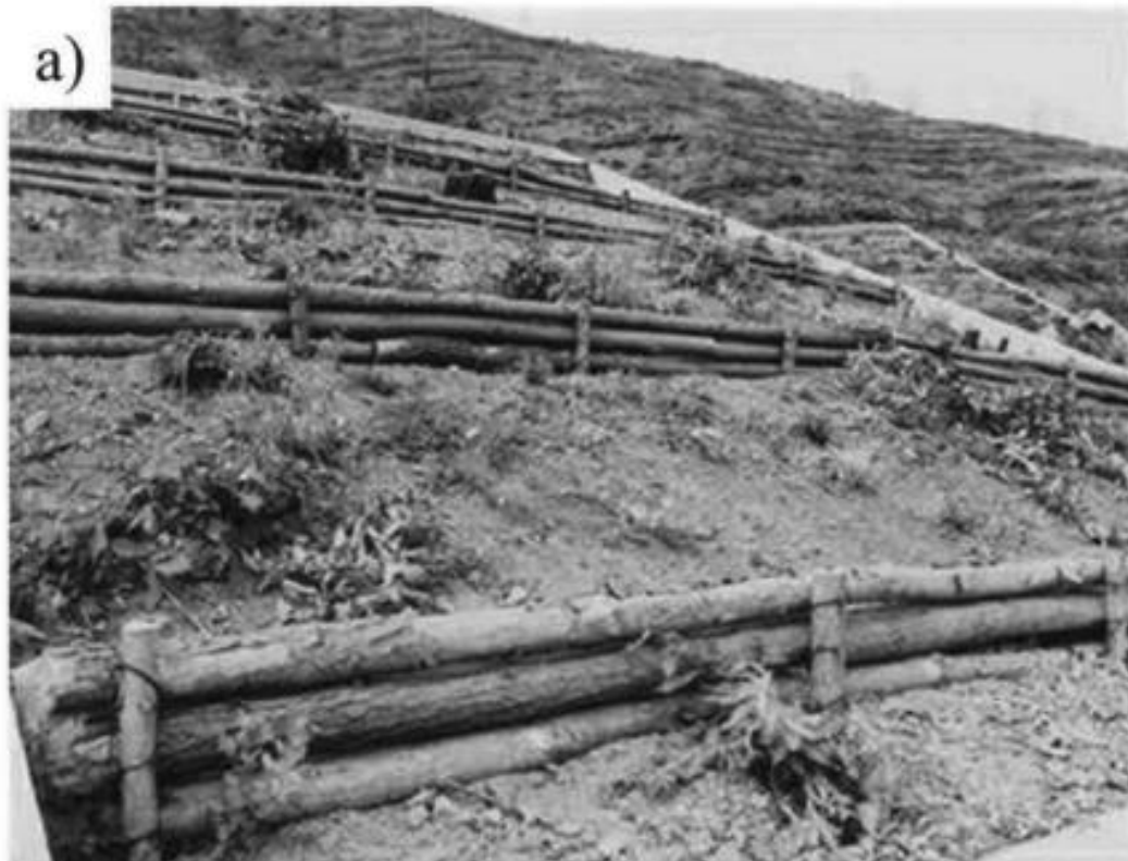
(a) Log strip terracing and (b) partially burned trees piling along a topographic contour in a burned area to prevent soil erosion
