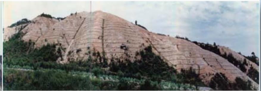
• Immediately after Restoration
