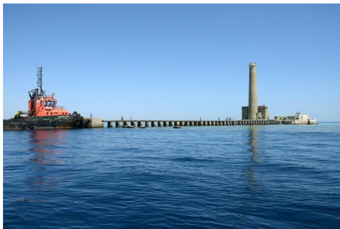
Fig. 1: The lighthouse and adjacent facilities (Photo by Hans & Nasr)
