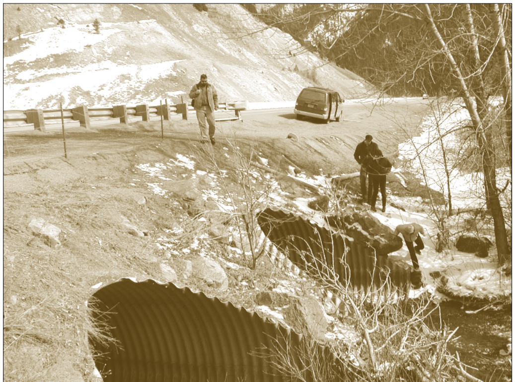
Culverts provide a wildlife corridor under Interstate 90 at Bozeman Pass. American Wildlands photo.
