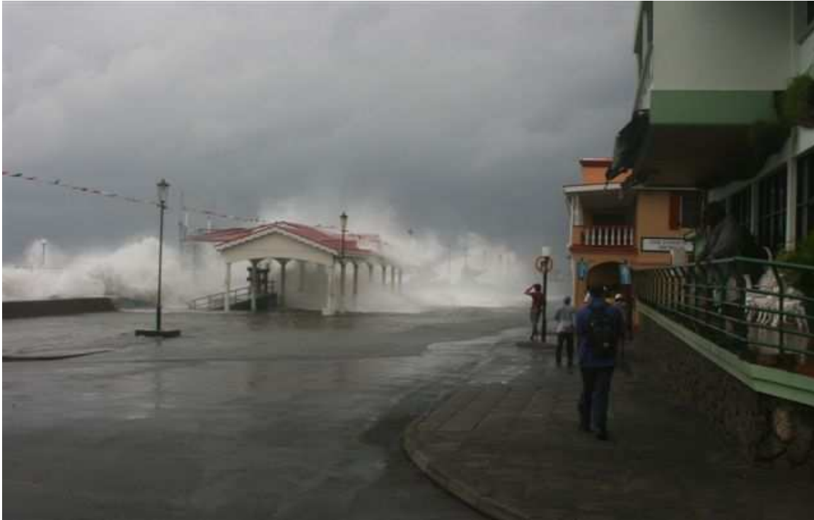
Figure 6 Wave-action during Hurricane Omar (2008) at the water front promenade, Roseau.
