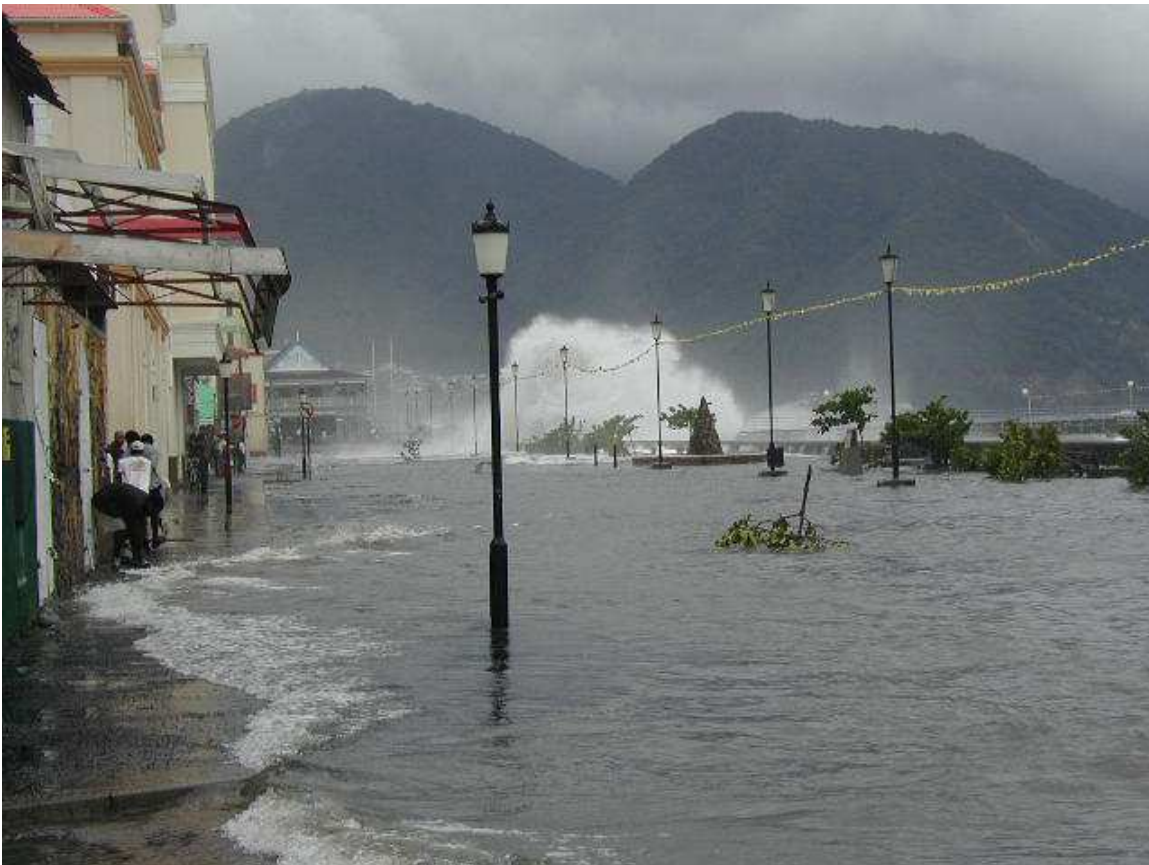
Figure 5. Storm surge of Hurricane Lenny in 1999 flooding the water front promenade, Roseau
