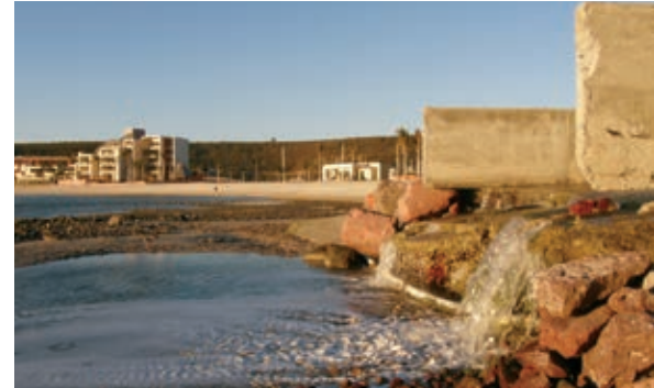
Many coastal properties have only rudimentary sewage treatment, or none at all. In coastal areas this leads to nutrient enrichment which can drive the formation of dead zones
