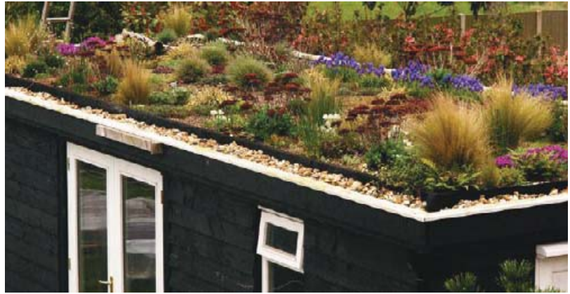
A green roof
