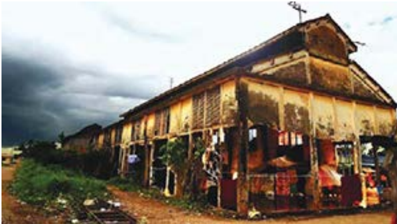
The rail yards and maintenance buildings
