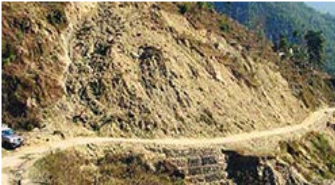
Slope stabilization methods were used for the Balephi landslide Source: Nepal District Road Support Program. www.flickr.com
