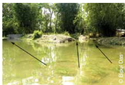
Step 5: Chanellizing the stream as necessary during the dry season for downstream water requirements.
