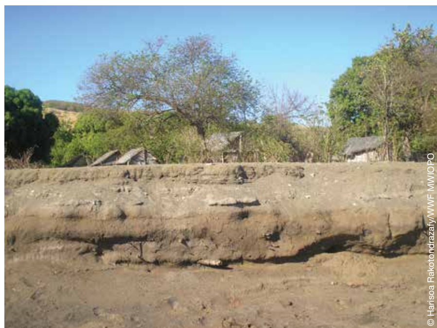
Coastal erosion due to sea level rise
