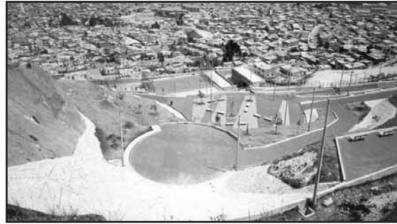
Side and top view of the Tanque El Volador Community Park. The water storage tank is a key structure in the water supply network.
