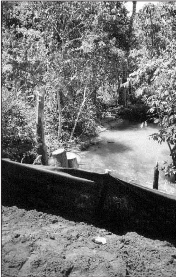
Sheet piling in conventional river crossings
