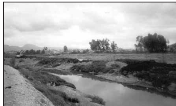
A typical canal, prior to the project, that posed a high sanitary risk, had poor environmental conditions and low aesthetic value.
