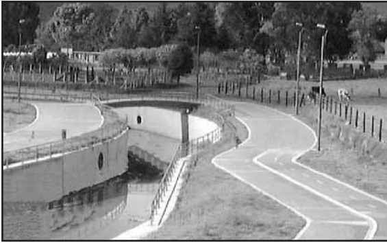
Torca Canal, after improvement of flow capacity and landscaping. Green slopes and fences around paths and bike trails on both sides of the canal significantly increased adjacent property values.
