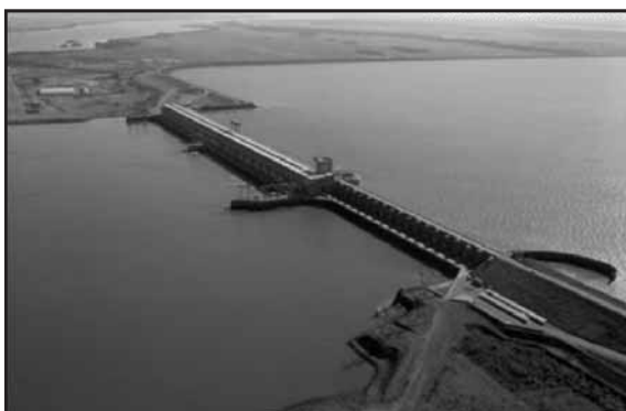
Aerial view of the main spillway at Yacyretá
