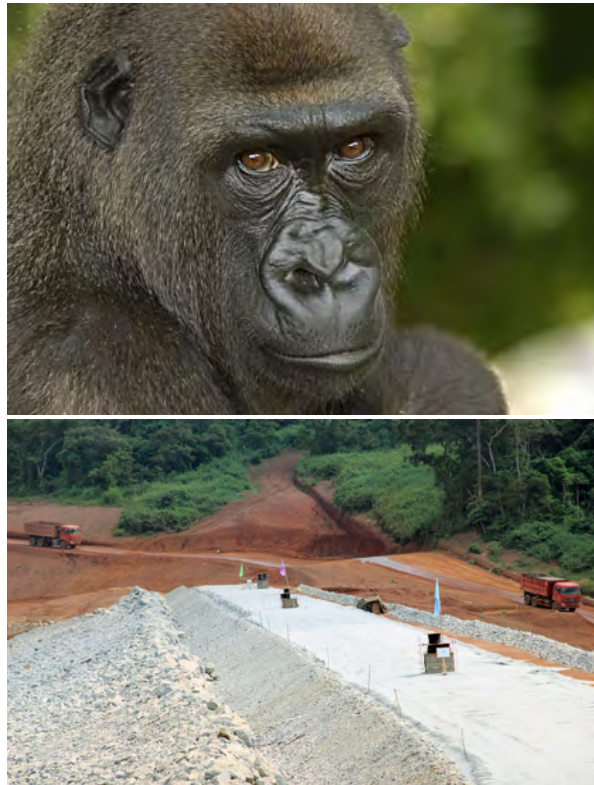
Western Lowland Gorilla Gorilla gorilla gorilla , one of the species protected within Cameroon's Deng Deng National Park, established as a biodiversity offset for the Lom Pangar Hydroelectric Dam project, shown here under construction.
