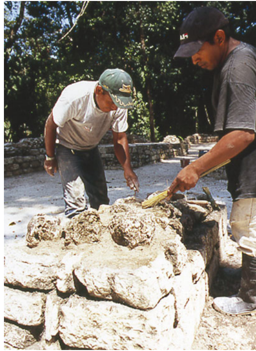
Masons occasionally experience a bad "mix," when the mortar doesn't cure properly. These workers had to dismantle previously restored walls and try again.
