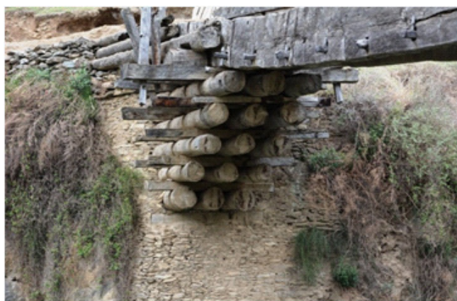
Stone walls fixed with black lentils and Bhojpatra
