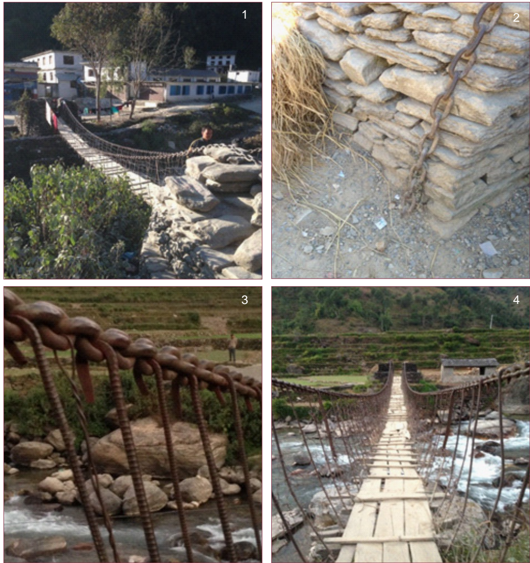
The chain bridges at Hatiya (Picture 1 and 4); The iron chain bearing the load of the bridge (Picture 3); The iron chain hooked into the ground (Picture 2)
