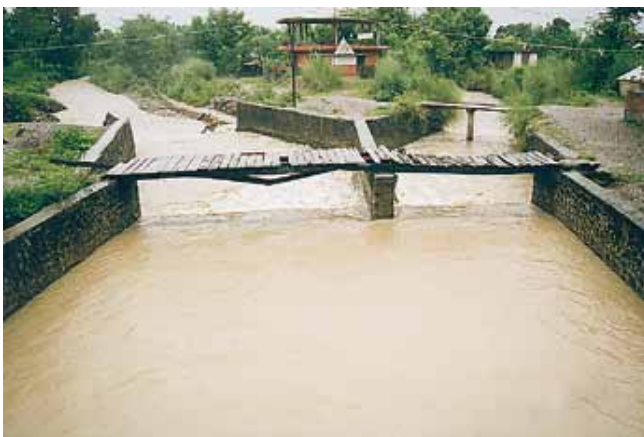
Tara Prasad Bhond: Locally made divider, 16-36 Mauja irrigation system
