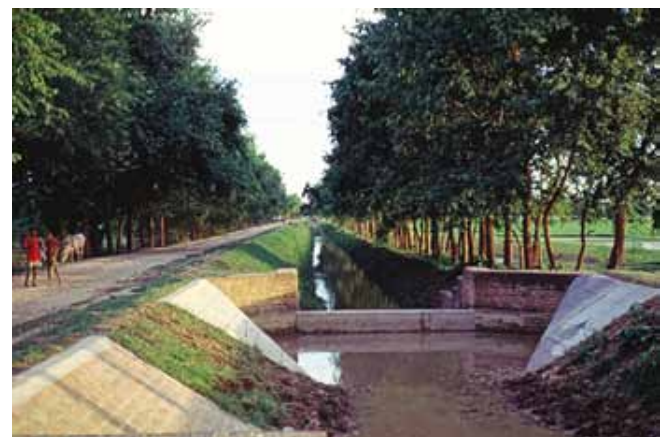
Marchawar irrigation system canal
