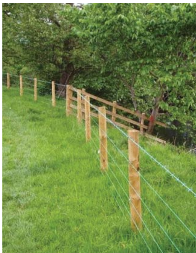
Fencing off of watercourses maintains the stability of banks and helps prevent erosion
