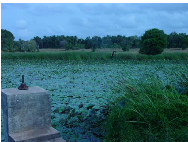
Picture 1: Small tank. Siltation is visible and is caused by soil erosion Courtesy: IUCN SL
